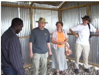
Half completed Kuku shed
